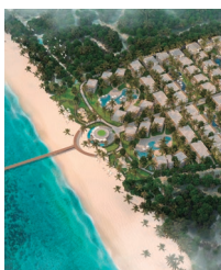
Corals of Zanzibar Beach Resort **** (Under construction)
