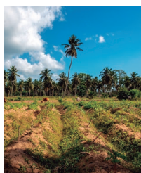
Pemba Farm Estate (Under construction)
